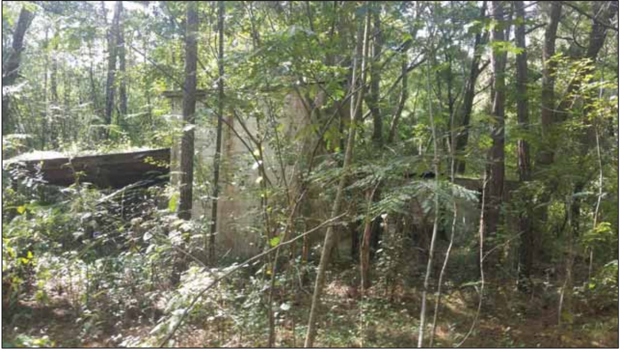
Figure 37. A dilapidated structure in the central areas of the study site.
