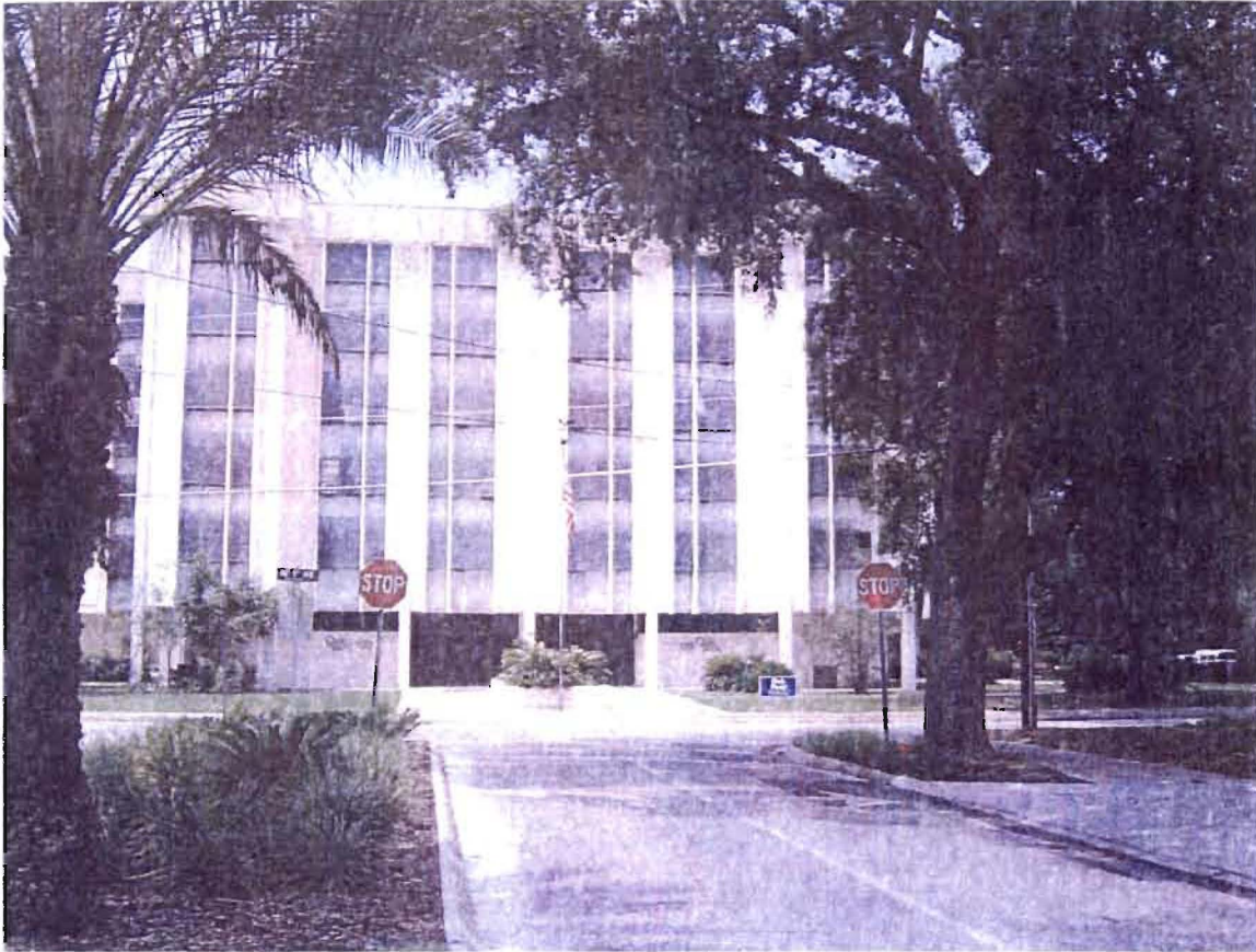
The existing Multi family complex across the street and to the north located on NE 8 th Avenue.
