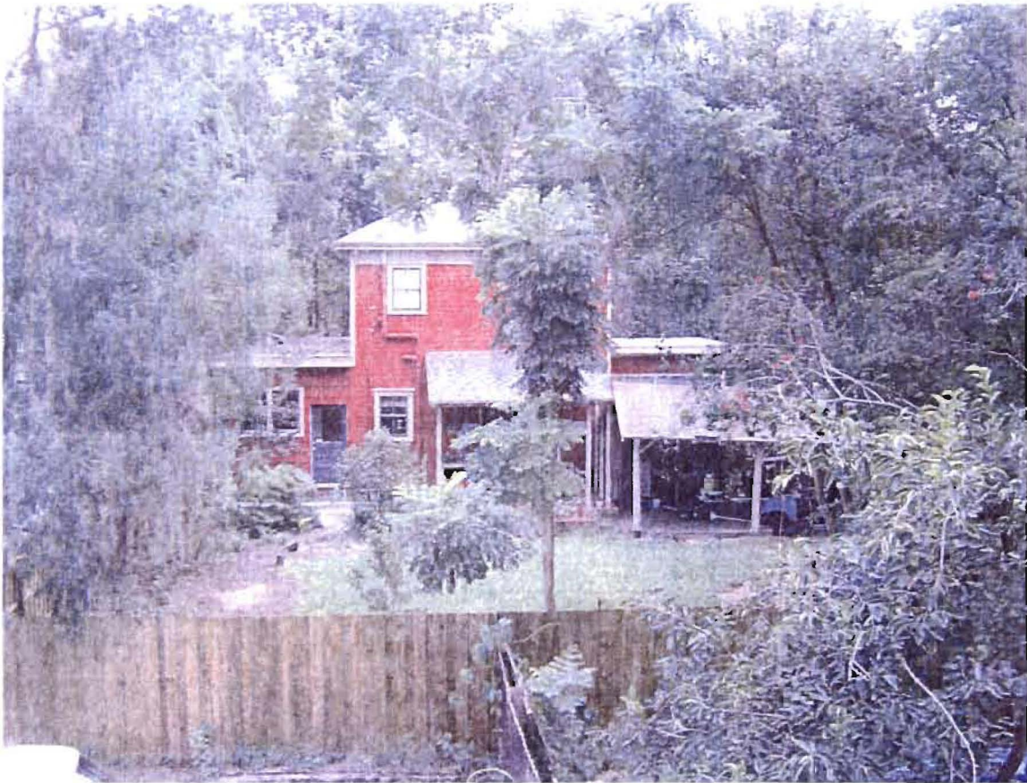
The existing residence to the rear of the proposed courtyard garden cafe area looking east.
