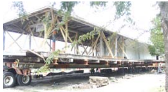
Depot building loaded on truck
