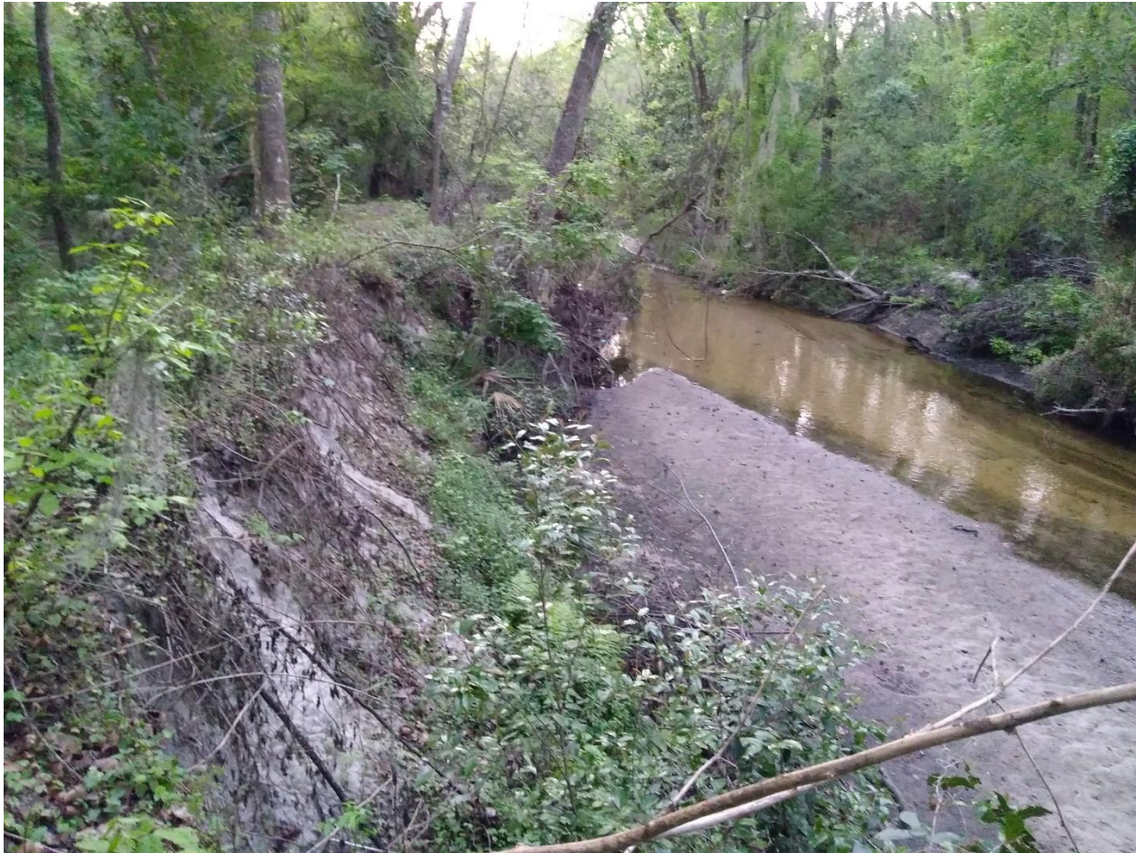
Photograph 17. Loblolly Woods, about 100 meters northwest of the western end of Northwest 11 th Avenue, near Florida Park, facing southwest on top of a constructed earthen embankment on the south bank of Hogtown Creek. The top of the embankment is about 5 meters above the bed of Hogtown Creek. The embankment is about one half eroded. Photograph by Wood in March 2018.
