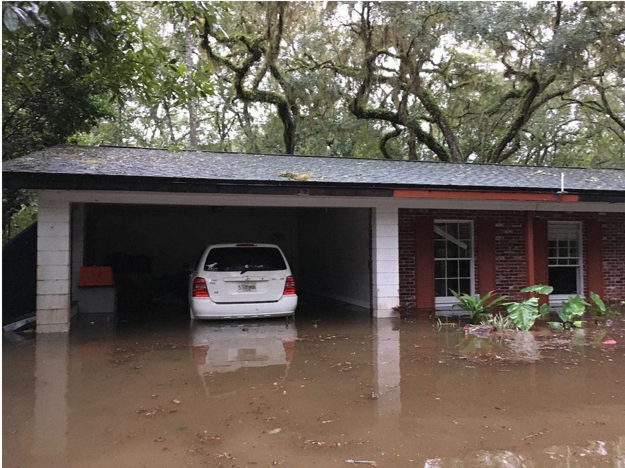
Photograph 1. Flooded house in Mason Manor, after Hurricane Irma, September 2017. Photograph from City of Gainesville Public Works database .
