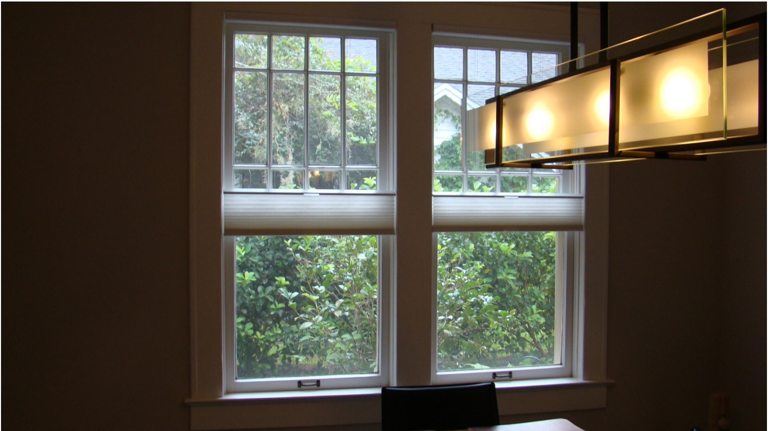
Original wood windows restored.
