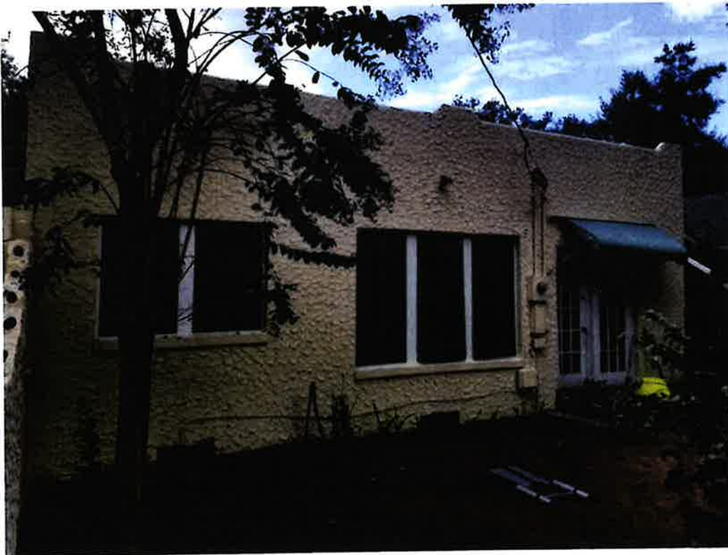
Photo of rear elevation
