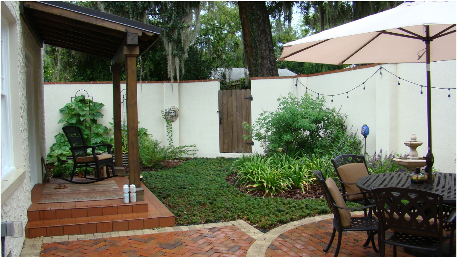
North view of Courtyard showing new porch and courtyard wall.
