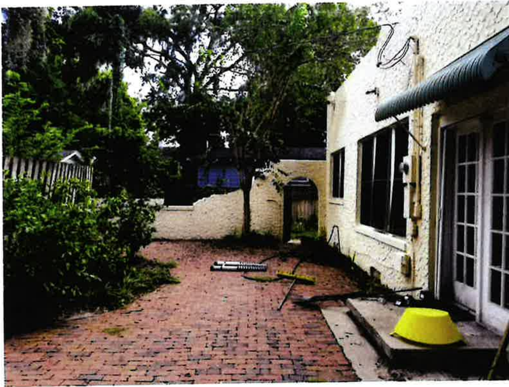
Photo (rear elevation looking South)
