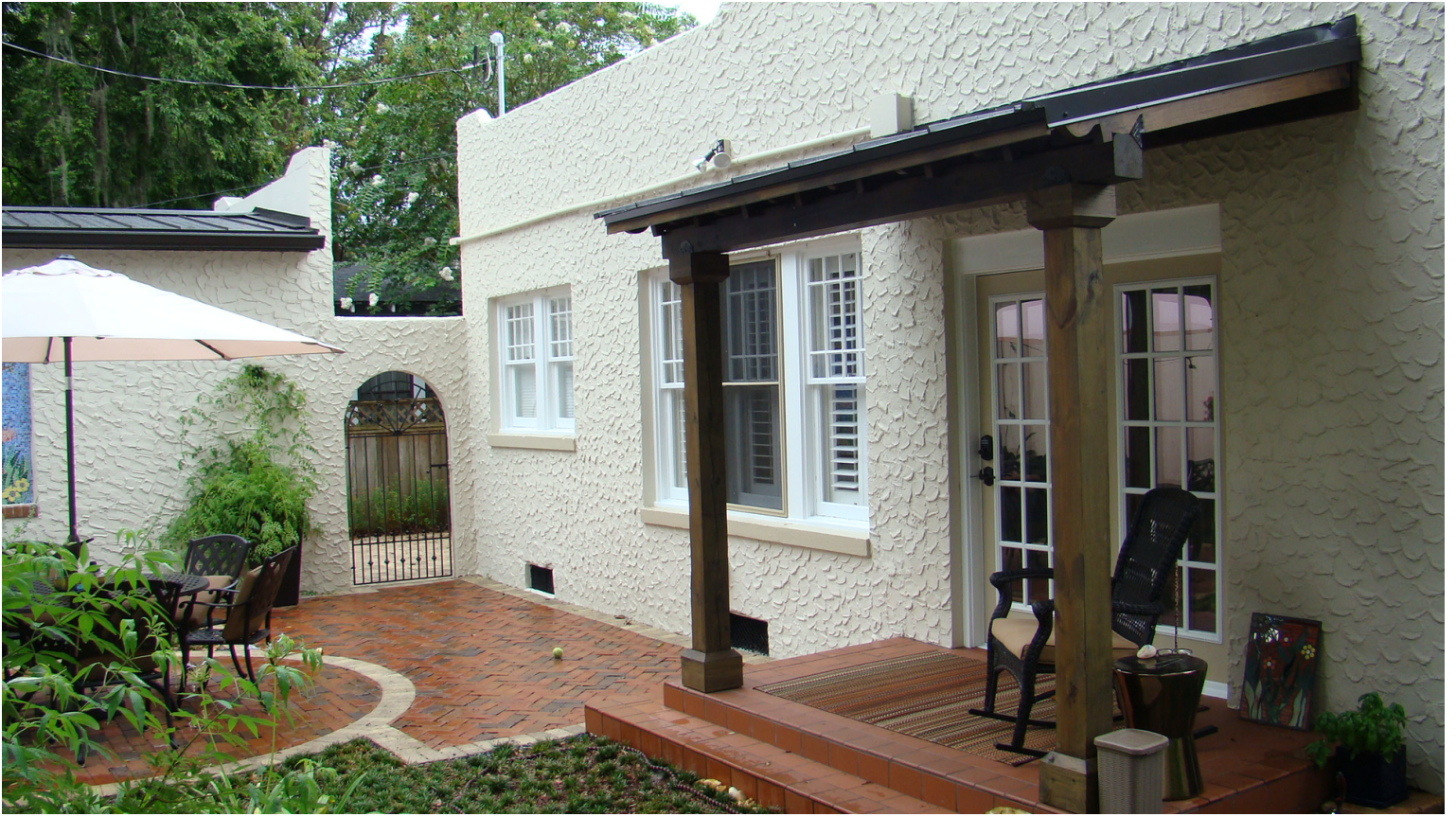
New rear porch, new rear garage to the left with only masonry arch saved from old garage.
