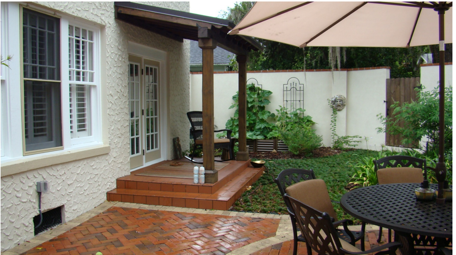
View of new rear porch and new courtyard wall and brick paving.
