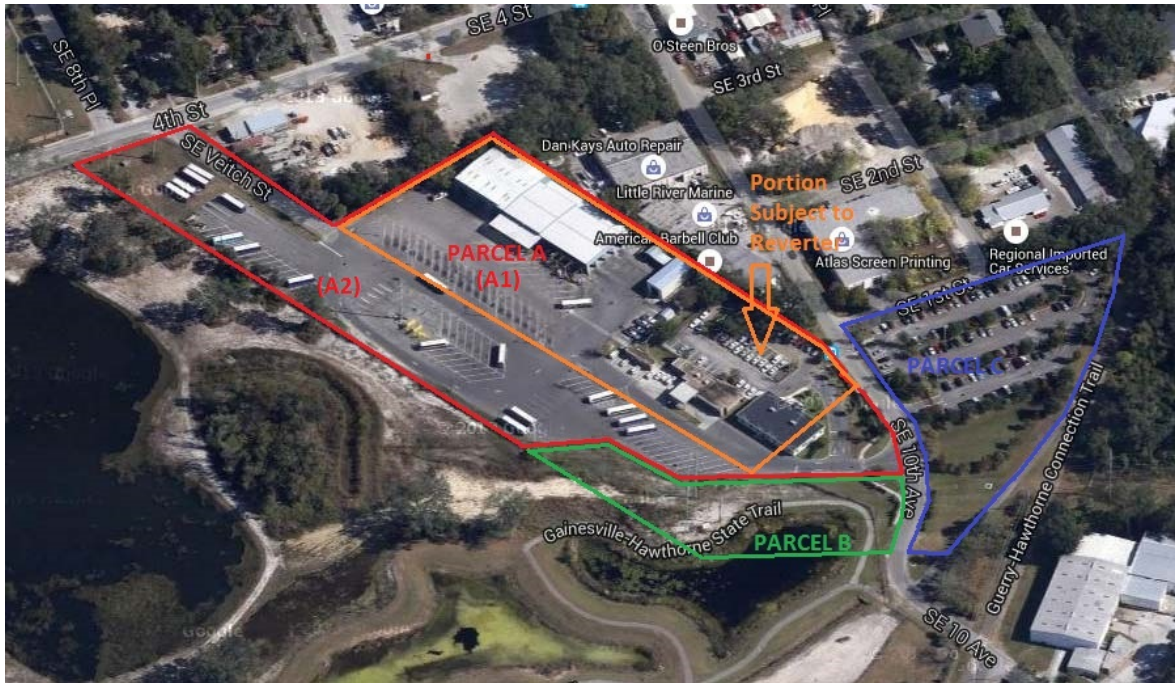
Figure1. - RTS Original Facility
