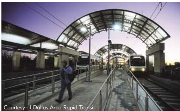
Courtesy of Dallas Area Rapid Transit
