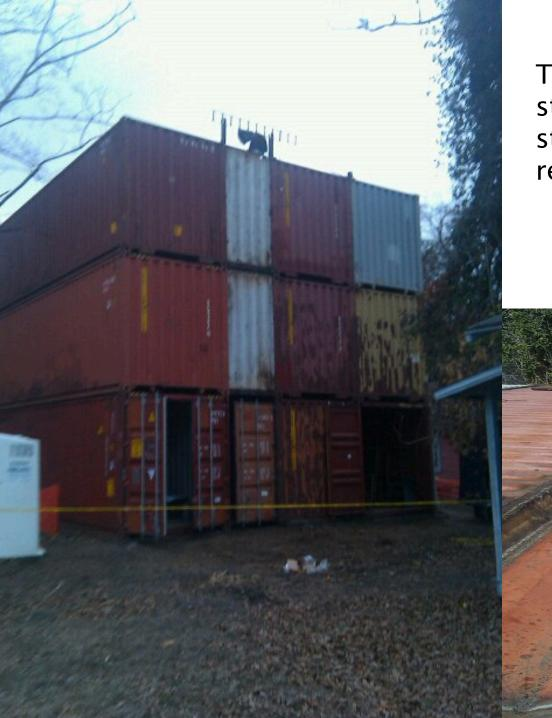
These are such durable structures built out of Corten steel, which is extremely resistant to rust.
