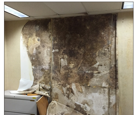
Mold Beneath Wall Coverings
