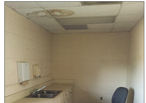
Water Damaged Ceiling Tiles
