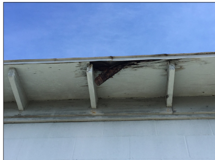
Rotten Wood At Roof Eave
