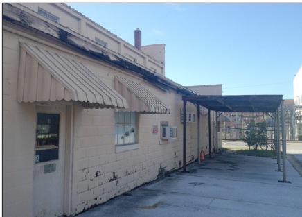
Deteriorating Exterior Paint On CMU
