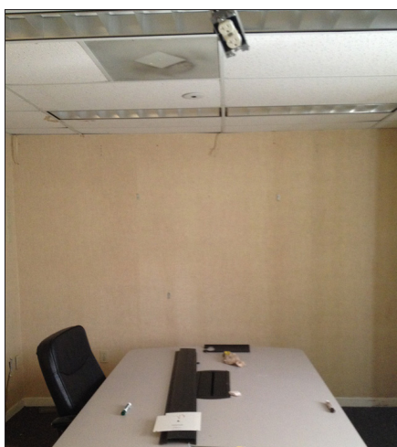
Electrical Components Hanging From Ceiling
