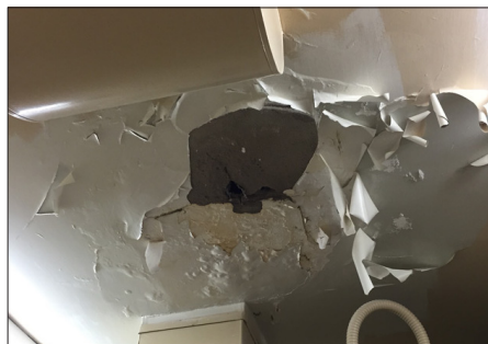
Water Damage Due To Roof Leak
