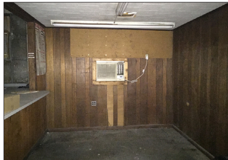
Deteriorating Interior Wall Finishes
