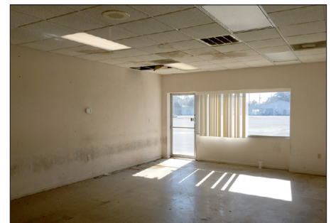
Water Damage And Mold Growth
