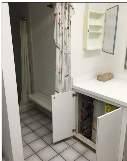
Toilet Room With Under-Counter Water Heater
