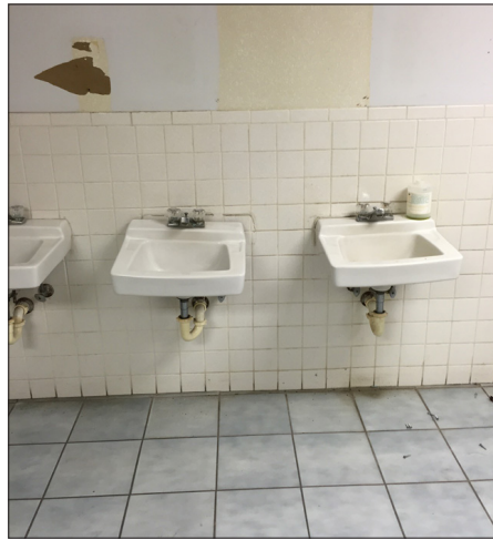
Water Damage At Sinks
