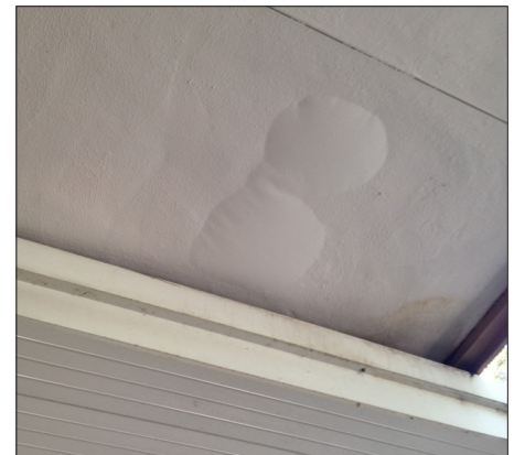
Damage Indicating Possible Roof Leak
