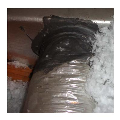
Reattached and sealed duct with mastic.
