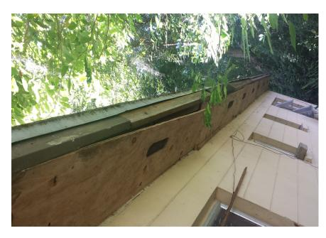
Necessary eave repair to prevent rodents from entering attic and damaging duct work and insulation.
