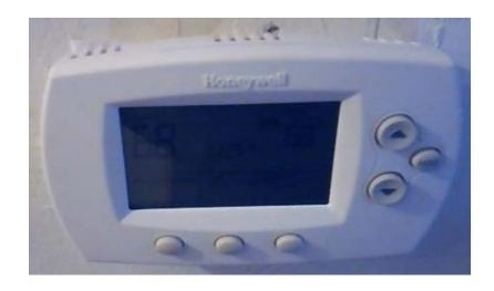
Replaced mercury thermostat with programmable thermostat.
