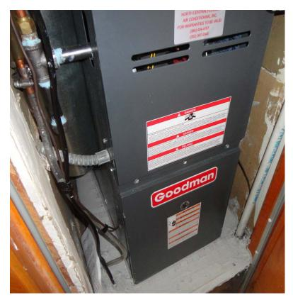
Replaced old, inefficient and malfunctioning air handler with new unit.
