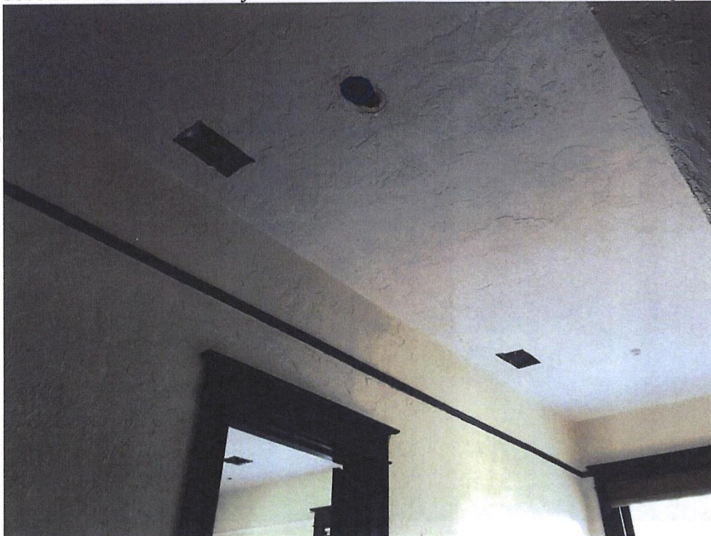
Second floor front hallway - Cut-outs indicate locations for two new registers
