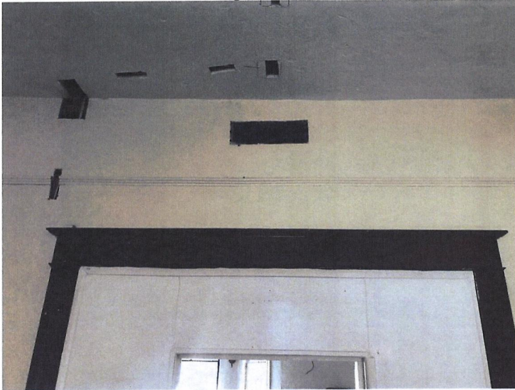
Parlor – Cut-out indicates new register location over doorway
