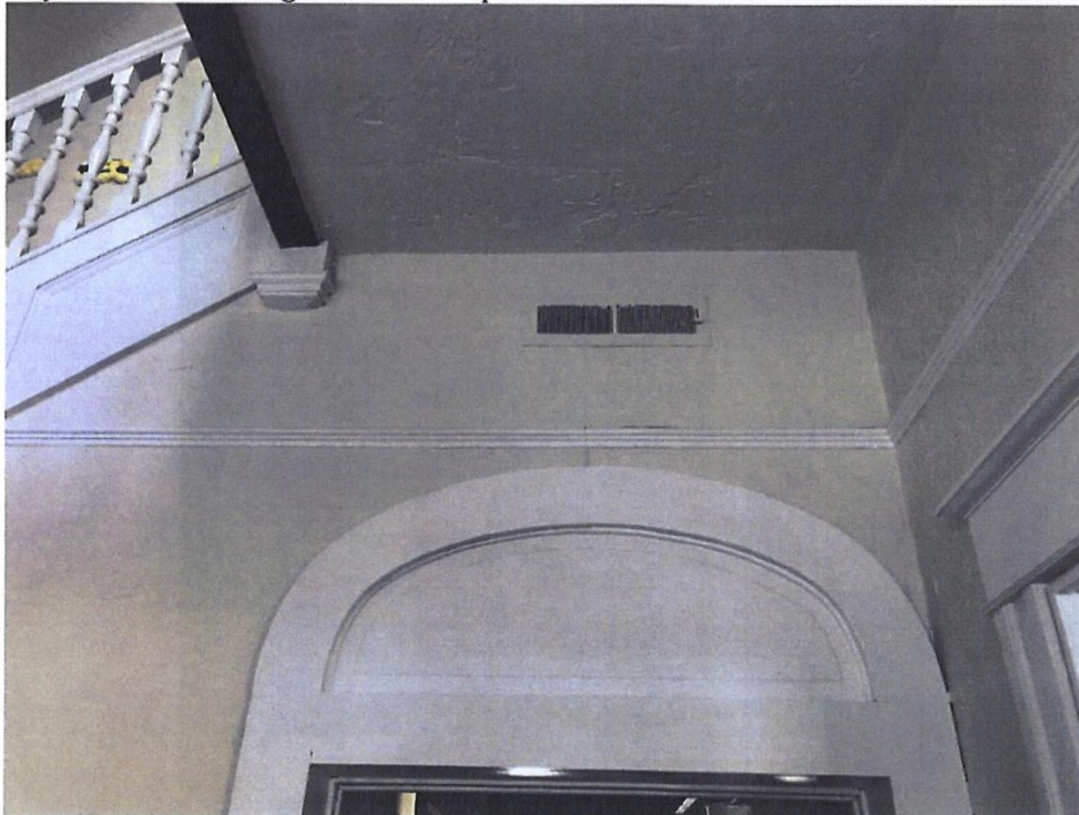
Foyer – New AC register will be placed at same location as old forced air vent
