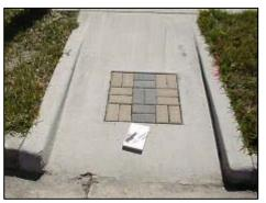
art. Construction of sidewalks and ramps can include such features as imprinting and brick or metallic inlays.
