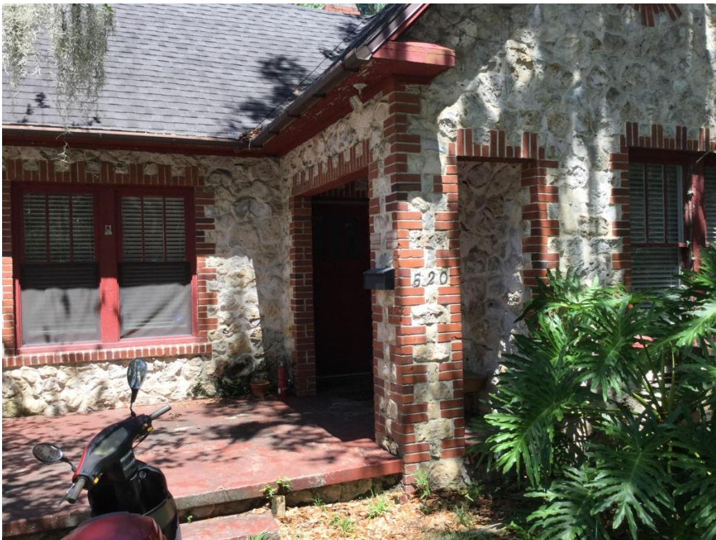
Top and Bottom: Details of front recessed entry to the right and raised patio to the left. The wood railing is not original to the house. The raised patio has a chert base and a concrete slab on top. 5
