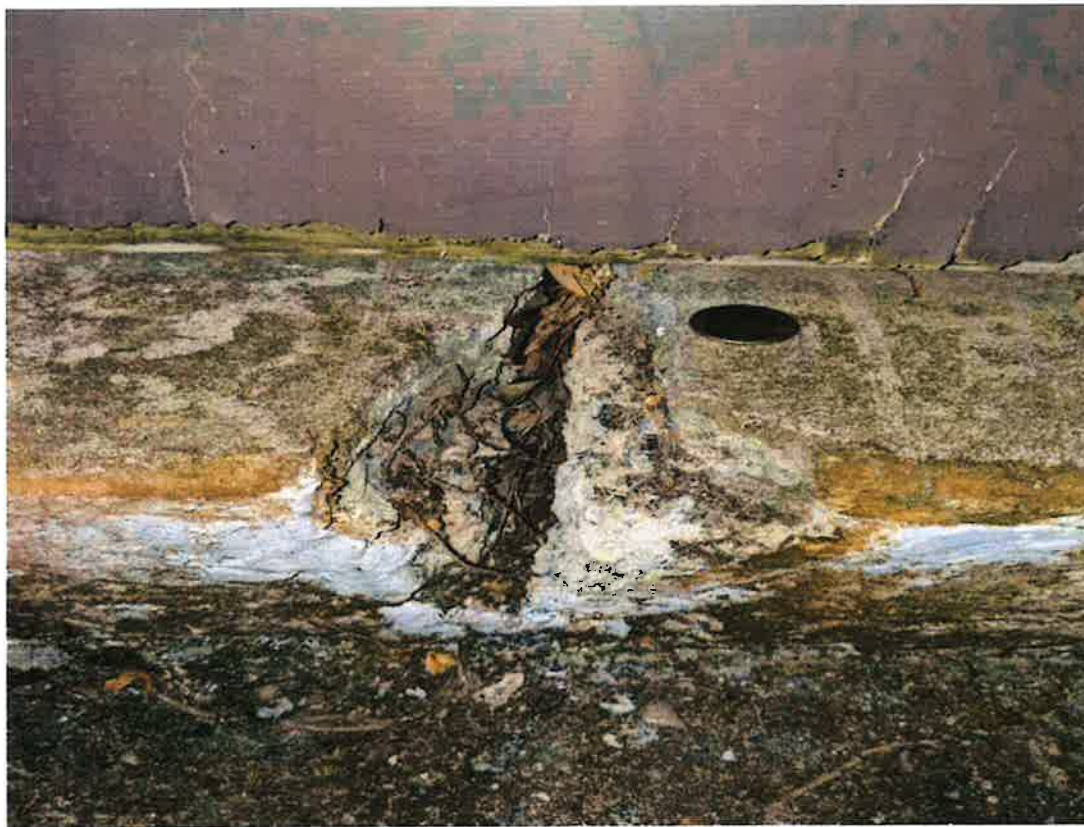
Structural slab crack
