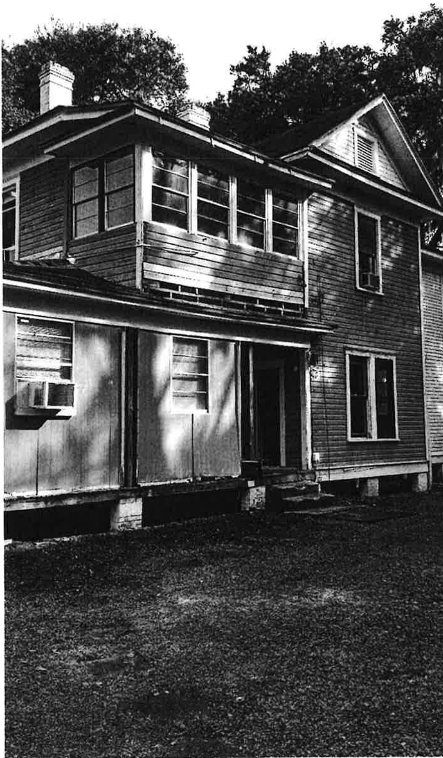
South Elevation, infill walls to be removed and porch restored.
