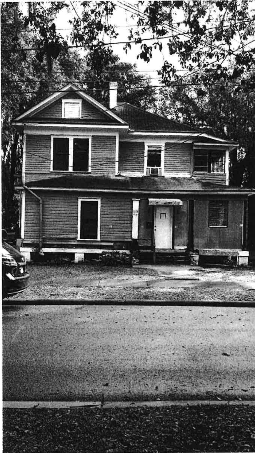
Front (West) elevation, infill walls to be removed and front porch restored.
