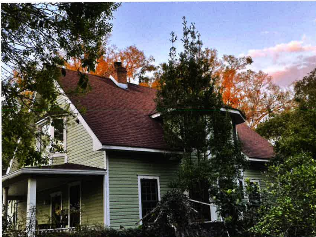
517 NE 4 th St, Gainesville FL 32601 - Reroof – Existing Roof photos
